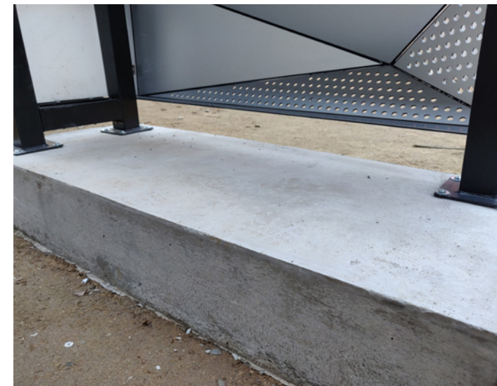
Concrete foundation smoothed with hand-trowel
