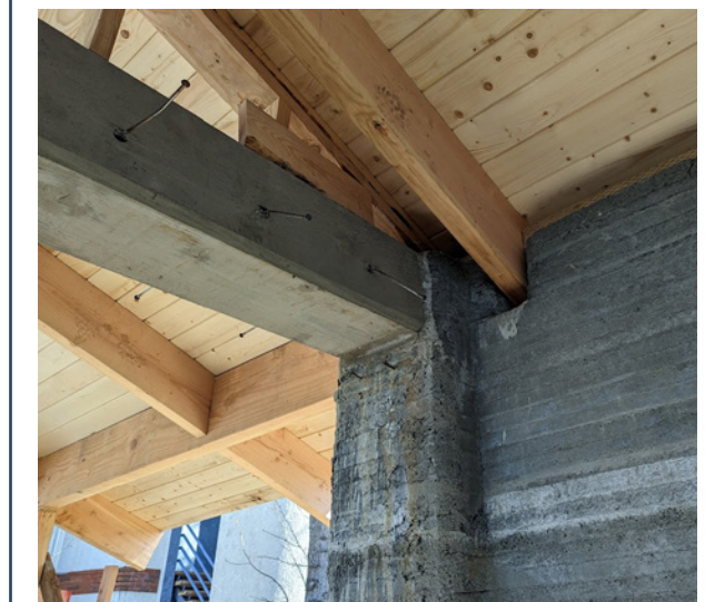
Slider header to 3D-printed column connection
