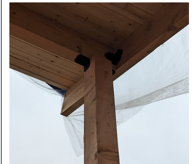
Porch post to beam connection
