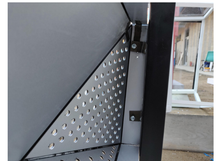
L-brackets connect panels to columns
