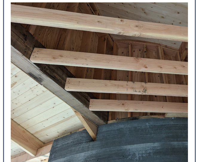
Pony wall to 3D-printed wall connection
